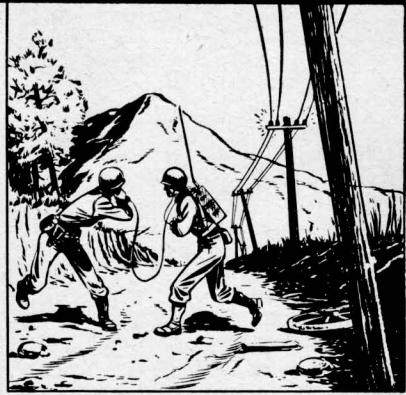
HIGH TENSION LINES
